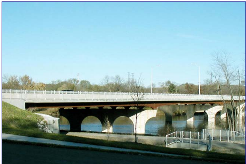
SULLIVAN ROAD BRIDGE AND BIKE PATH
