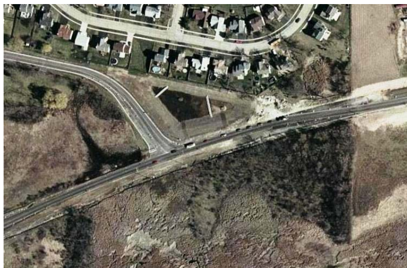
CONSTRUCTION OF HOOK ROAD RELOCATION AT ROLLINS ROAD.
