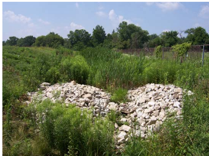
DIVERSION CHANNEL WITH RIFFLES AND POOLS AND NATIVE PLANTINGS.
