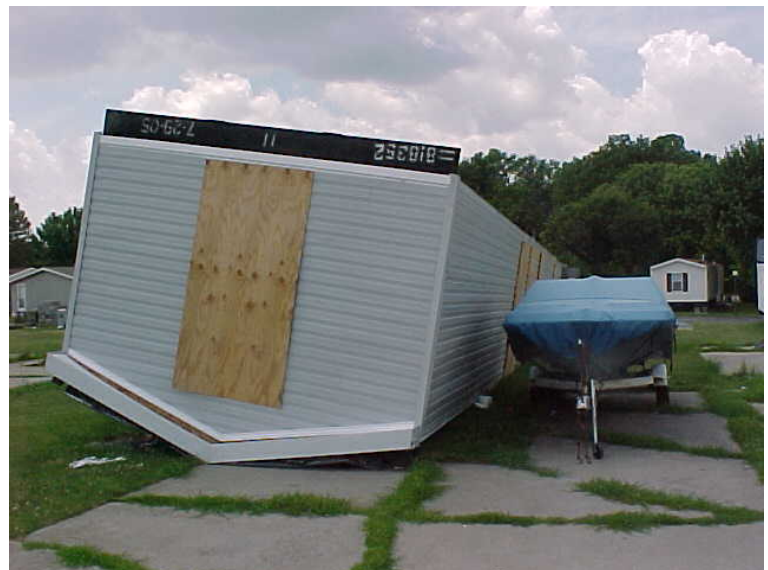
ANCHORAGE AND TIE DOWN INVESTIGATION
