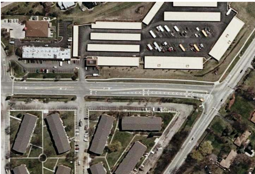
BUTTERFIELD ROAD BUILT FOR FUTURE EXPANSION WITH DUAL LEFT TURNS.
