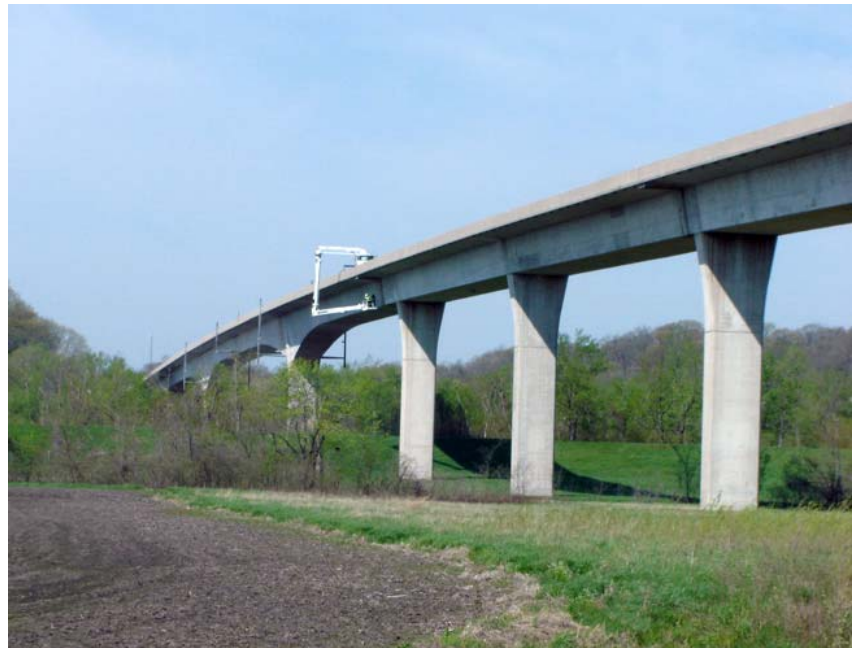
EAST BOUND I-72 STRUCTURE INSPECTION
